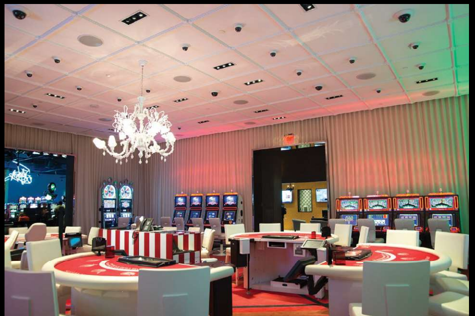
Speakers are set up in two zones in this room designed to provide an exclusive gaming experience for patrons. Local sources including a DJ can be inserted at control points in the gaming pit.
